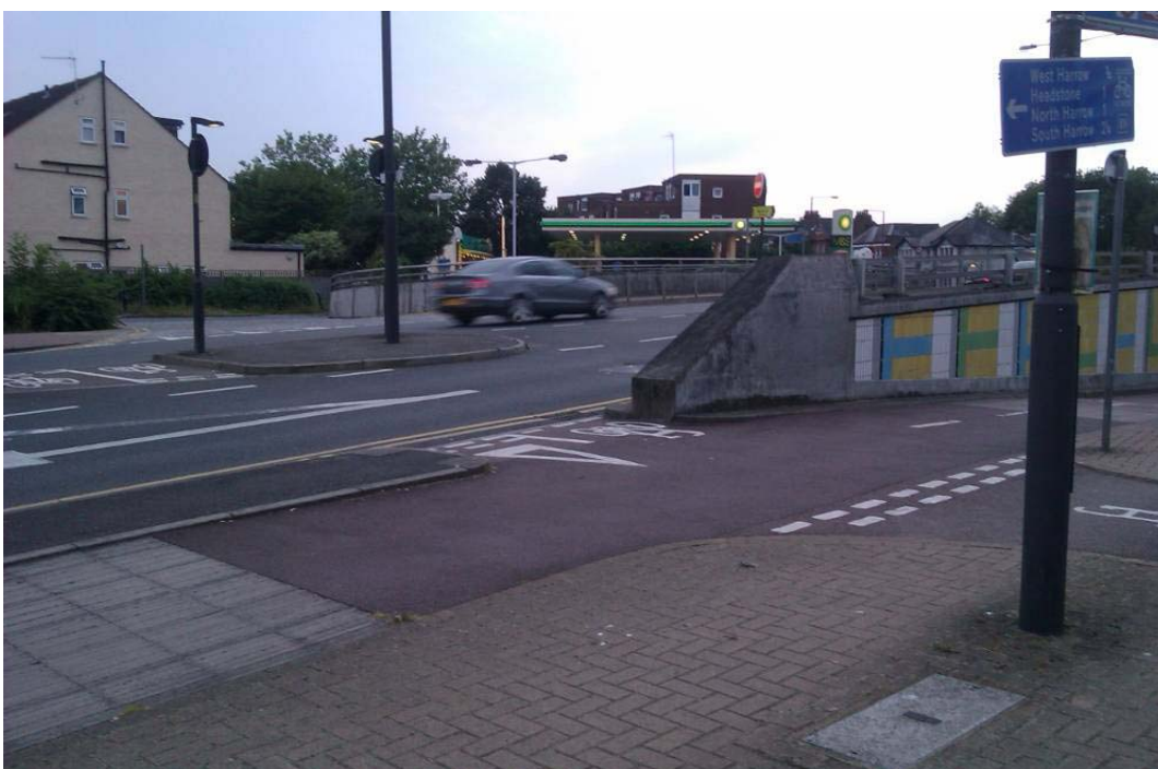
Subway entrance at the Roxborough bridge roundabout
